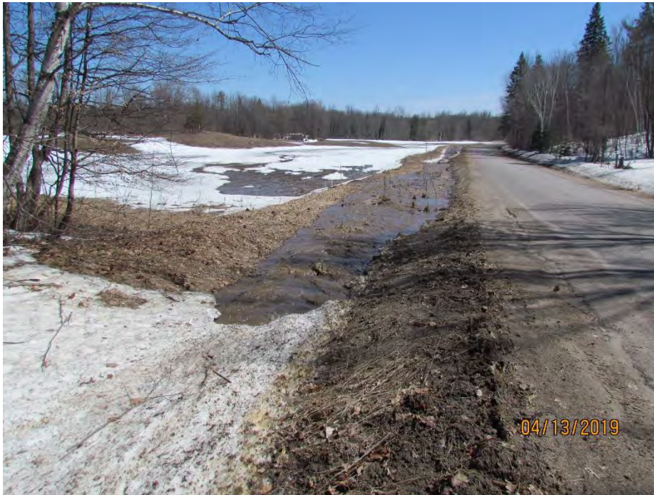
Photo 11 (Looking S): Station 8+300 – The east side of Ferguson Lake Road, showing significant drainage path and management issues.
