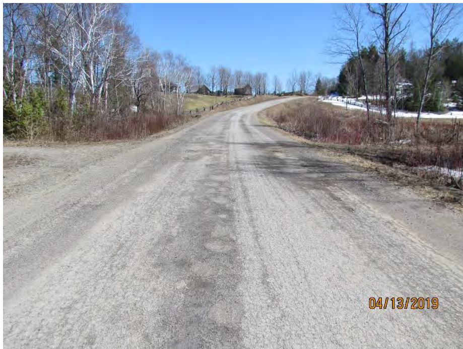
Photo 10 (Looking S): Station 7+000 – Typical poor road condition section showing various cracking types and depressions, potholing and multiple repairs.
