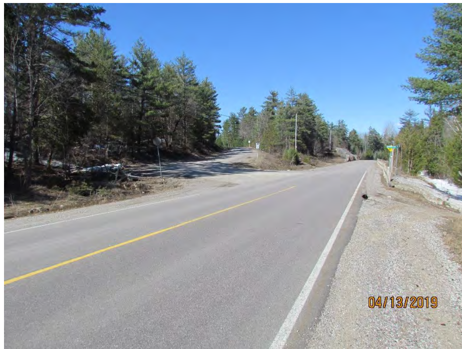
Photo 2 (Looking NE): Station 0+000 - Intersection of Calabogie Road and Ferguson Lake Road, showing adverse intersection geometry, absence of hazard signage, etc.
