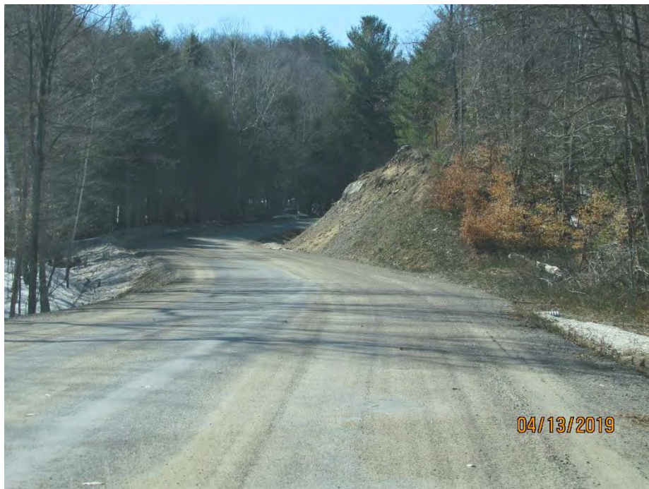
Photo 8 (Looking N): Station 4+000 – Ferguson Lake Road, high bedrock area and steep slopes on east side of the road.
