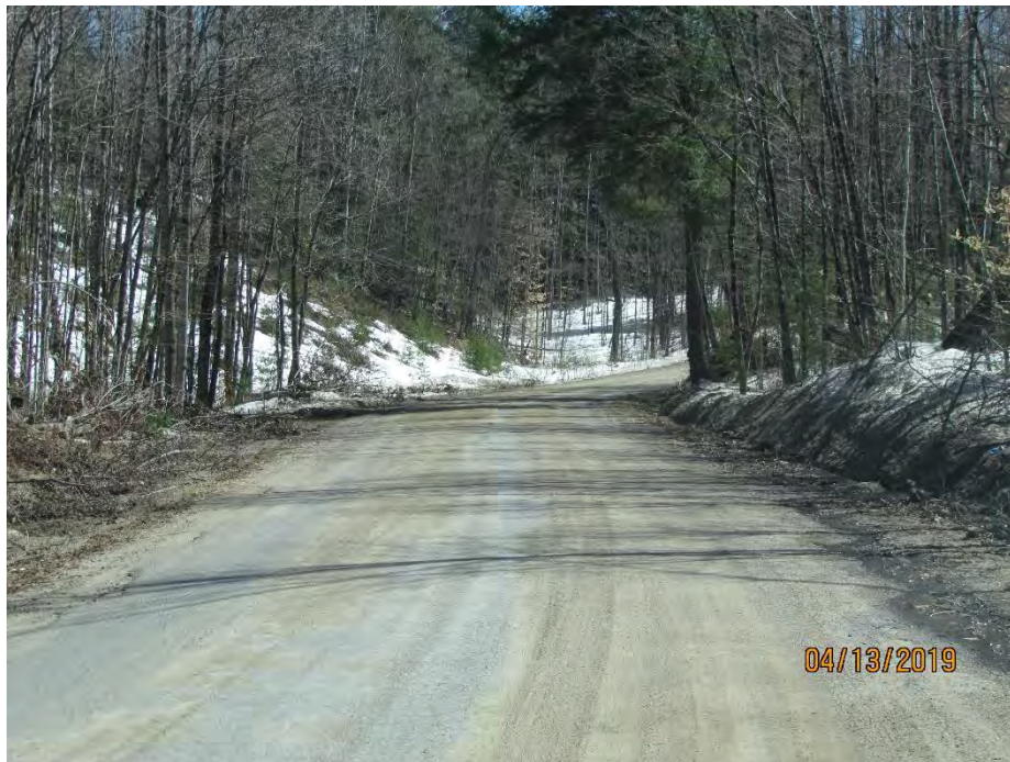
Photo 3 (Looking W): Station 1+300 – Going down Ferguson Lake Road towards the tornado affected area, showing vegetation encroachments, minimal road width, drainage deficiencies, and deteriorating road conditions.
