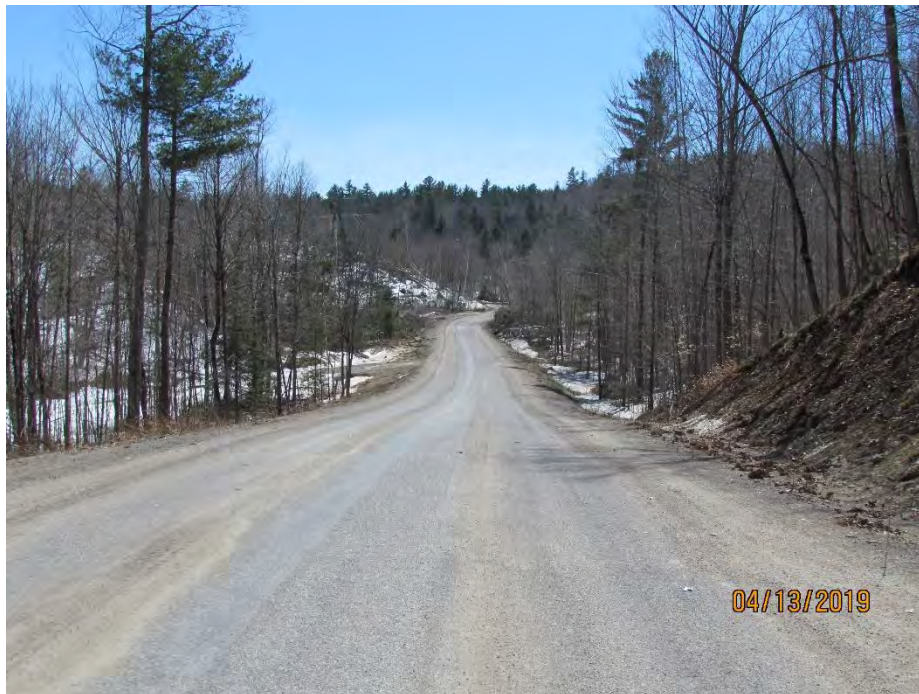
Photo 7 (Looking S): Station 1+650 – Area in need of horizontal and vertical re-alignment, road widenings, and drainage management/measures.
