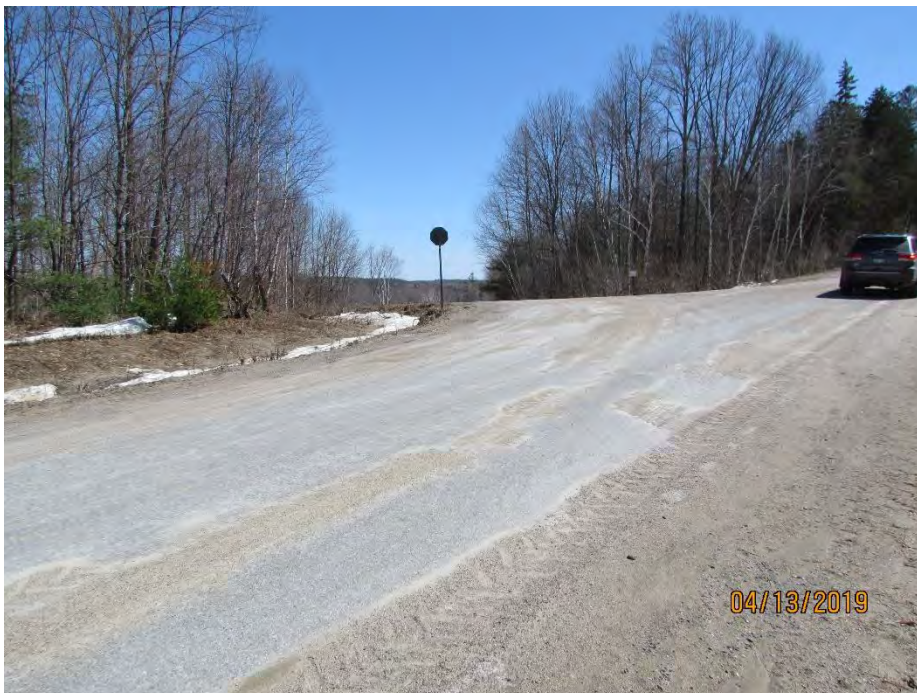
Photo 12 (Looking S): Station 8+500 – At intersection of Kennelly Mountain Road and Ferguson Lake Road, showing obstructed sightline with vertical alignment.
