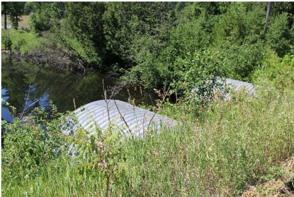
Plate 8: Double corrugated metal culvert located between Kellys Road and Constant Creek.
